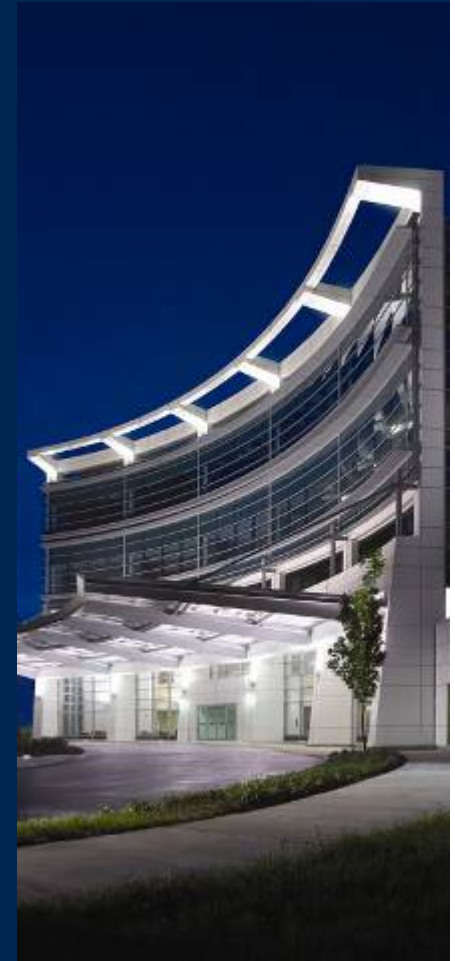
Chippenham Medical Center, Virginia
