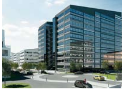
The 12-story Havneholm Tower will be a new landmark in central Copenhagen, Denmark. With about 18,500 sq. m. (199,000 sq. ft.) of leasable space, it will be completed in 2010.
