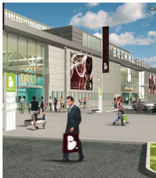
A 1947 aircraft hangar will soon be a 3-story retail space at 45,000 sq. m (484,000 sq. ft.) Bromma Center.
